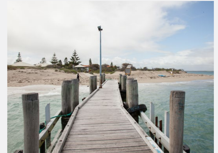
Photo 23A: Jetty at Mersey Point.
