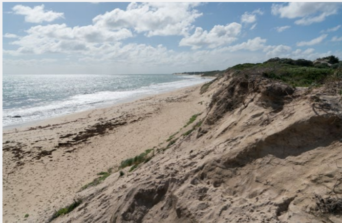
Figure 59: Beaches adjacent to wild connectors are generally accessible, although often through informal beach access paths and prohibited means such as 4WD.
