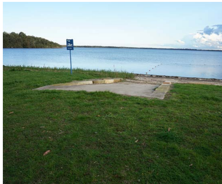
Figure 16: A small ramp at Tom Burke Reserve provides vehicular access to remove wrack, and could also be used for launching boards.
