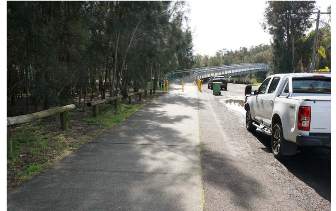
Figure 12: Pedestrian bridges ensure the continuity of shared paths despite watercourse inlets, such as this one over Saltwater Creek.
