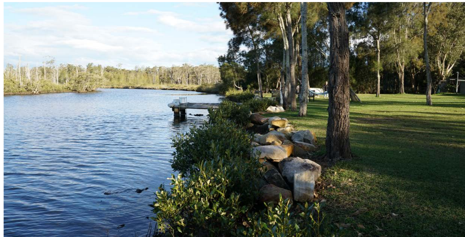
Figure 25: Looking south along Lloyd Avenue Local Connector to the mouth of Karignan Creek.
