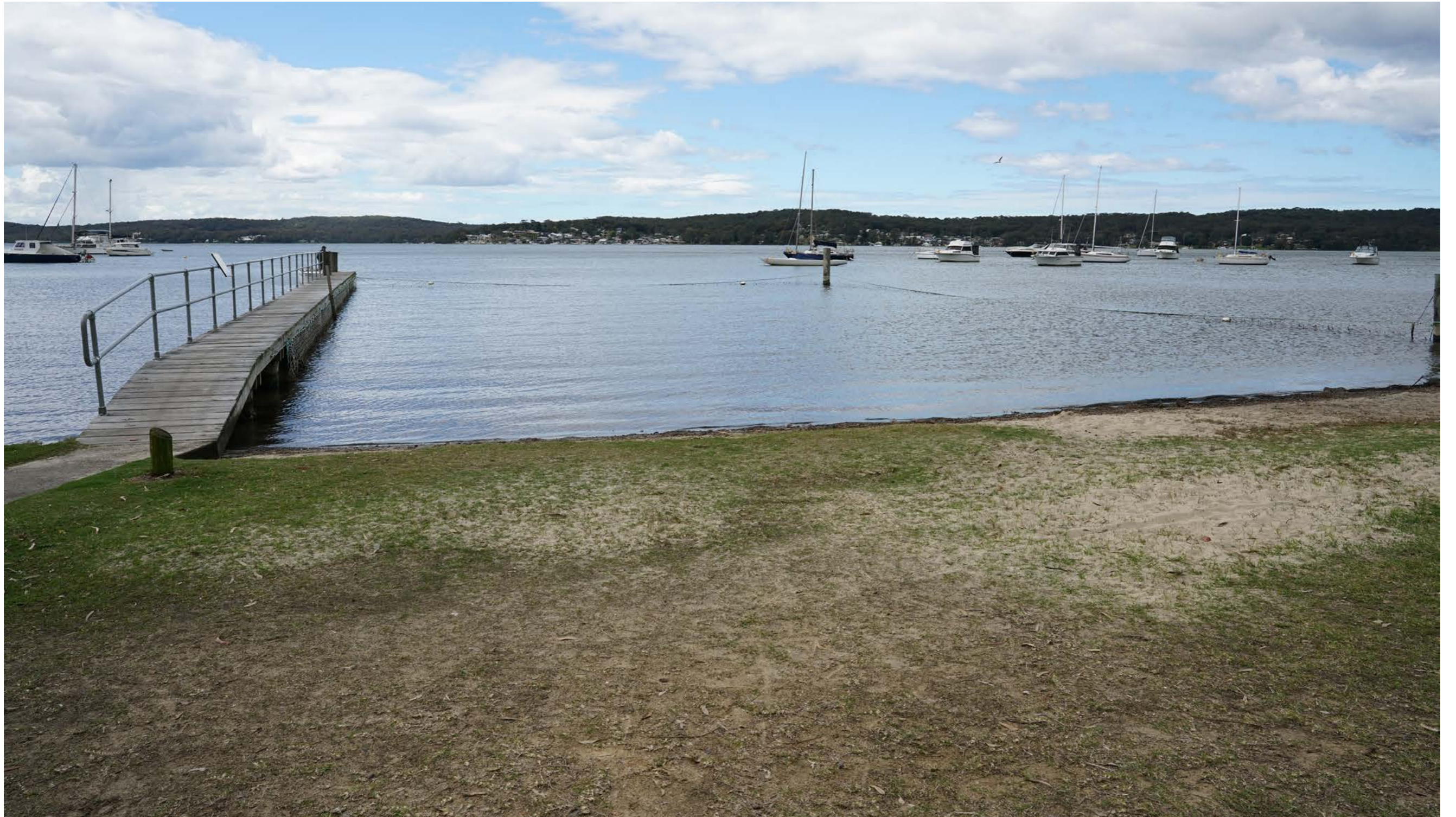
Figure 36: Jetty and swimming net at Gwandalan Lioness Park.
