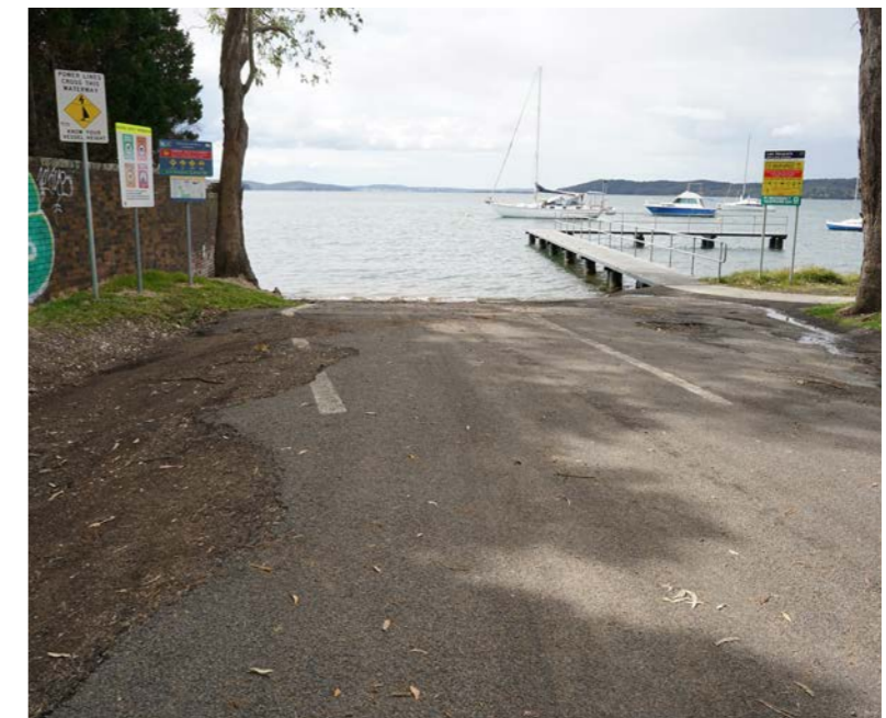
Figure 33: Garema Road Boat Ramp.
